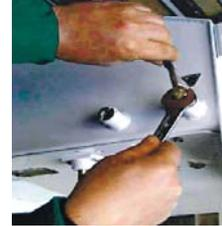
The outdoor switching module is earthed by means of an M12 hex head bolt (provided) threaded into a captive thread on the back wall of the tank. The RC (ILC) cubicle is earthed by means of an M12 hex head bolt (provided) threaded into a captive thread on the base of the cubicle.
