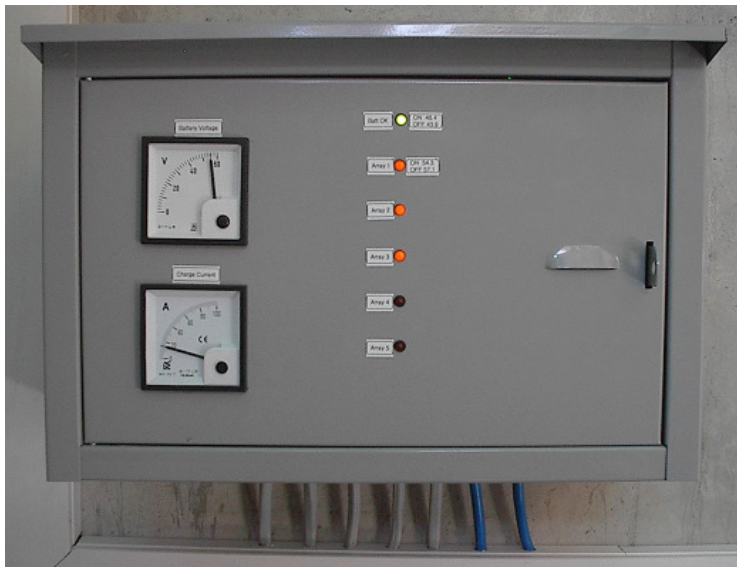
Figure 9 Front of the charge regulator
