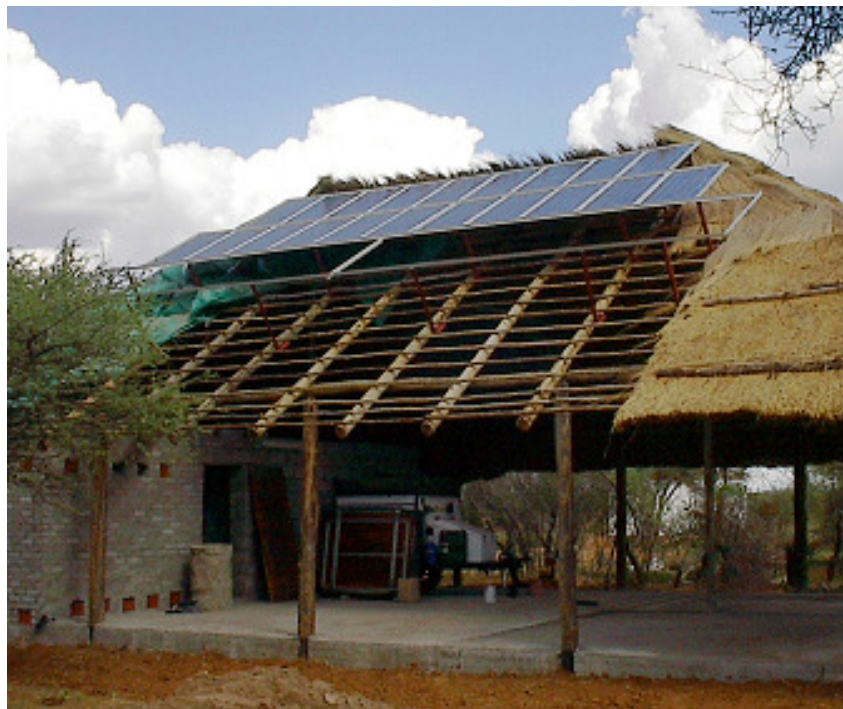
Figure 4 Layout of the solar panels on the roof before thatching
