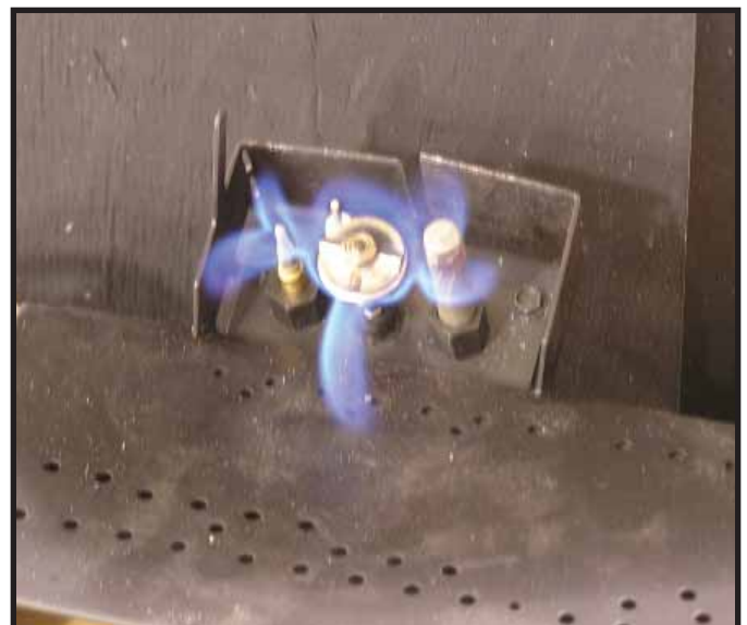
Figure 3.1 Standing Pilot Flame Patterns
