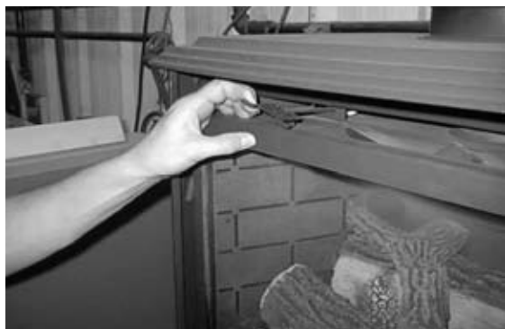
Figure 17 - Removal of Sealed Glass
