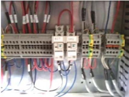
One of these relays is operated by the Bitronics, the other by the cDAQ. Both are triggers for the safety circuit. The terminals to the left are the connections to the safety circuit, and the terminals to the right are the connections to the Hall effect sensors located in the DC disconnects.
