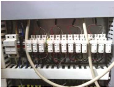
These relays are the interface for the digital input signals for the Summit® DC supply. The supply interprets certain pins in the user cable shorted to a common return pin as digital inputs. The digital outputs from the cDAQ operate the relays to perform the shorting action. There are six relays for each half of the supply.
