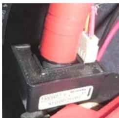
These are located on the positive DC lead in the DC disconnects. They provide a direct measurement of the DC bus current that is sent to the analog input module in the cDAQ.
