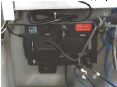
The control PC, monitor, and the Linksys hub are plugged into the battery backup ports on the UPS. The supply for the cDAQ is plugged into a surge suppression port. This way, loss of the 120V source removes power to the cDAQ, which triggers the safety circuit.
