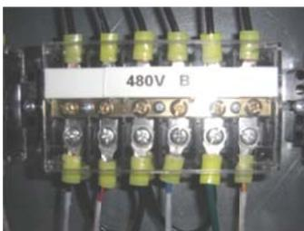
The shorting blocks provide a location to short together the CT leads. This provides an added measure of safety if the metering configuration ever needs to be altered later, as open CT leads can develop extremely high voltages.
