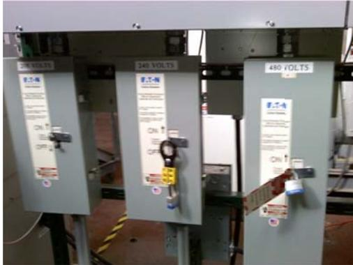
These are the points of connection to InteGrid and the main AC supply for the simulator. The shunt trip modules are activated by the safety circuit to isolate these sources from the simulator.
