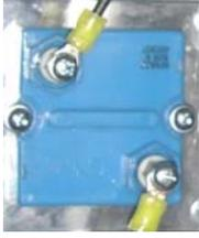
These resistors provide the preload required by the Summit® DC supply. There are five resistors wired in series, with the whole string connected in parallel with each half of the DC bus.
