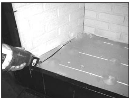
Figure 12.2. Using a saws-all, cut out the floor.
