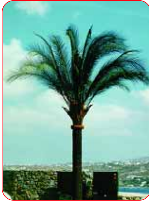
Base station blended into the environment in Greece
