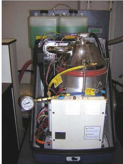
7. Once the pressure is checked and confirmed to be at the correct level, leave the pressure gauge attached to the WhisperGen™ as it will be required again later in the commissioning process.
