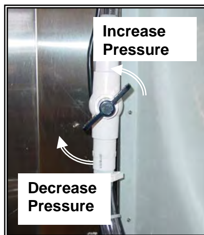
Adjust Water Flow 18", 24", 36" & 48" PolarCool
