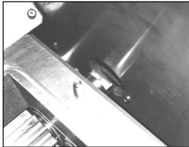
Hopper pump drive shaft alignment
