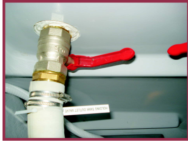
Waste water tank discharge valve
