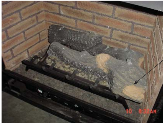
Figure 48 - Placement of Log 2
