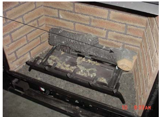
Figure 47 - Placement of Log 1.
