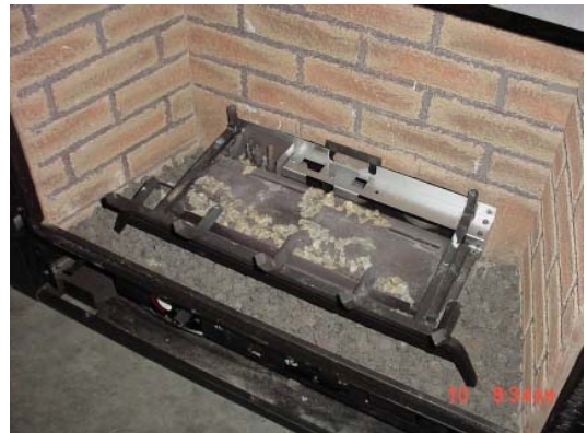
Figure 46 - Placement of Rock Wool on Burner
