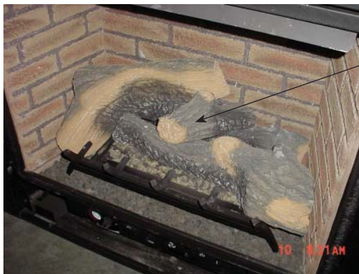
Figure 50 - Placement of Log 4
