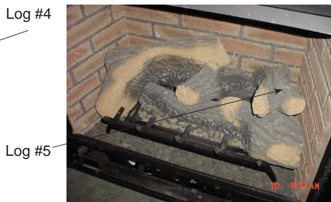
Figure 51 - Placement of Log 5
