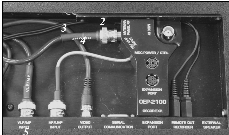
Figure 4 INSTALLATION OF THE OEP
