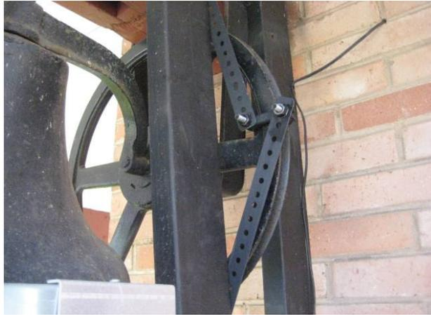
Connect the rope wheel clamp to the perforated steel straps to anchor the bell in position to the frame. **Use Loctite or Gorilla glue on the clamp's threads.**
