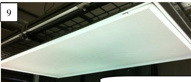
9 Close lens, turn on circuit breaker and energize the fixture.
