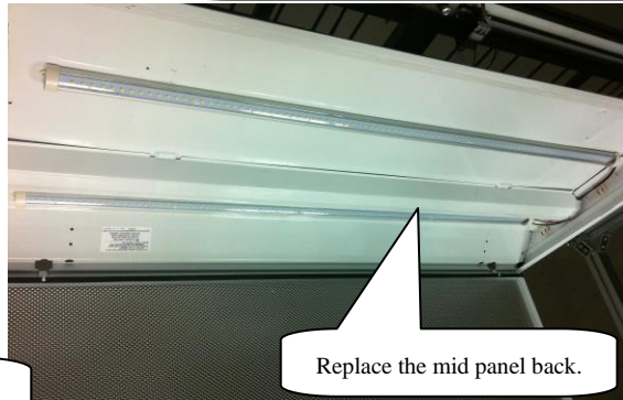
7 Secure the ends of the LED tubes with self-drilling screws. Place the Magnetic Tubes into the fixture. Connect the LED driver to LED tubes using quick connectors.
