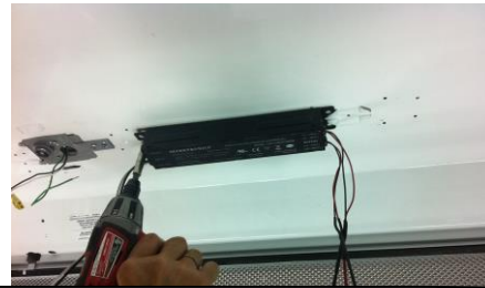
6 Attach quick connectors to the inputs from the new LED Driver and secure it to the fixture with the original screws.
