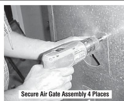
**Figure 13 - Install Screws**
