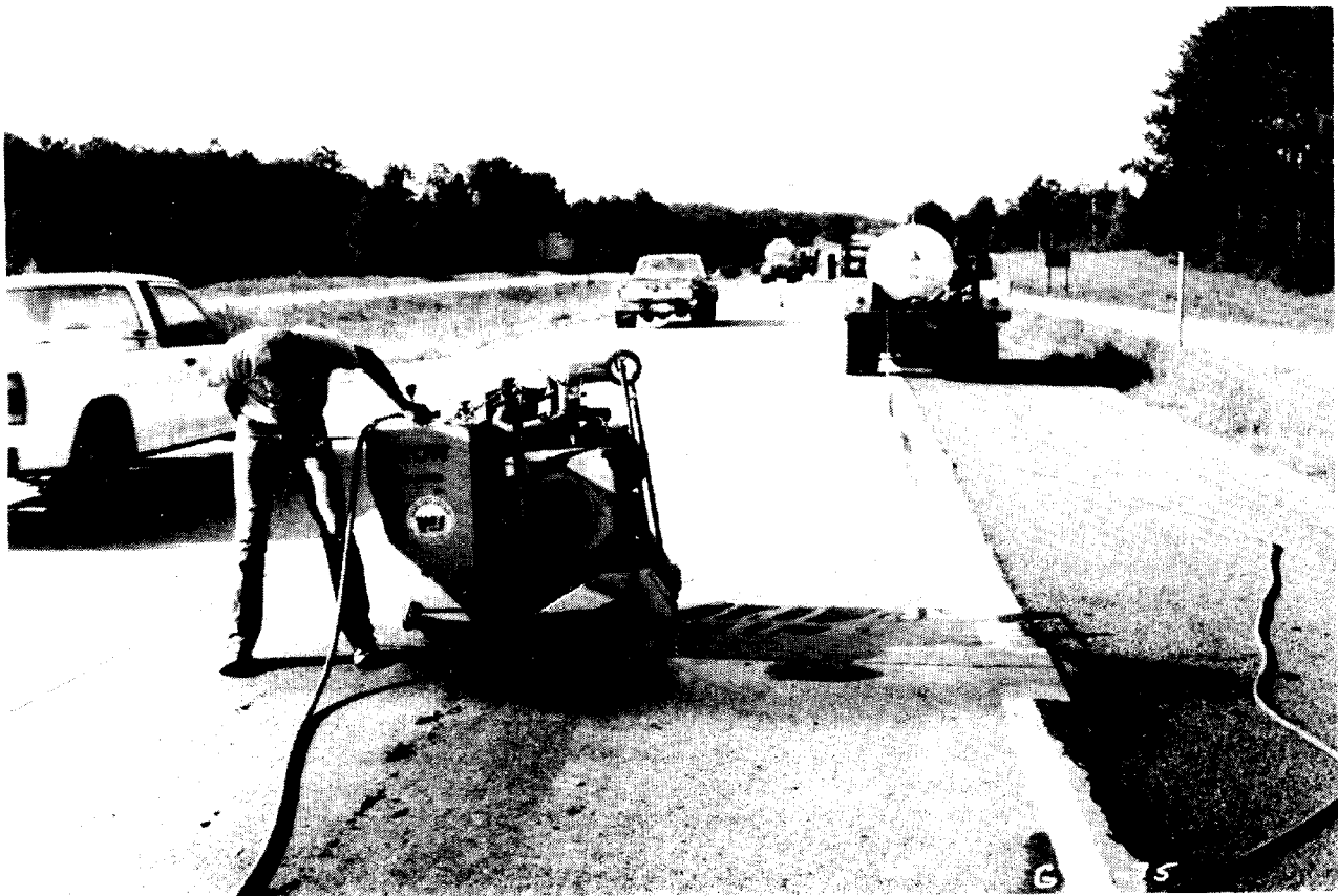
Figure 4-1. Concrete Saw Refacing Joint.
