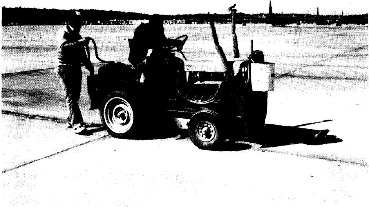
Figure 4-3. Joint Plow Removing Old Sealant.
