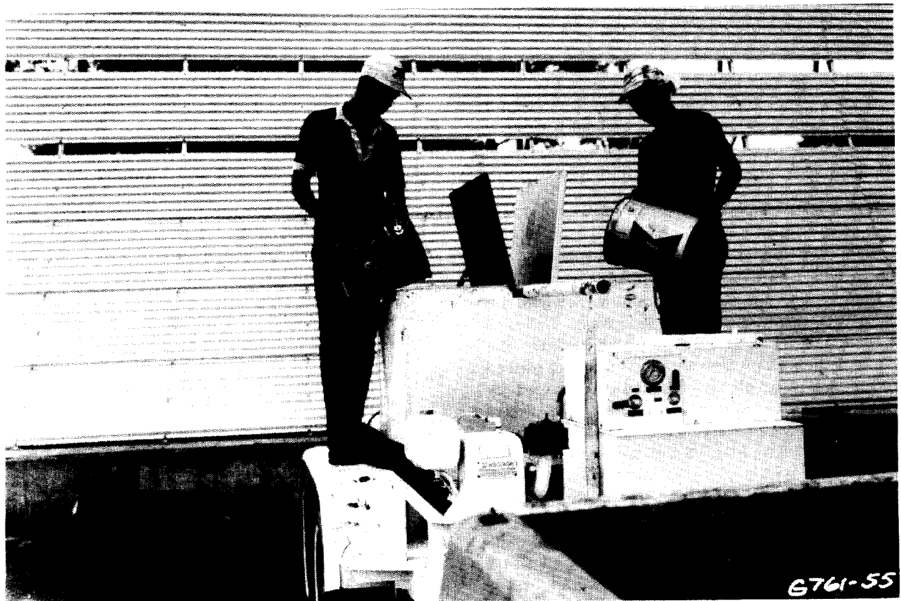
Figure 5-3. Cold-Applied, Two-Component Sealant Application Equipment.
