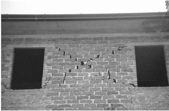
Compression-bending failure:
