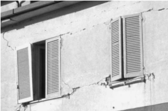
Compression-bending failure:
