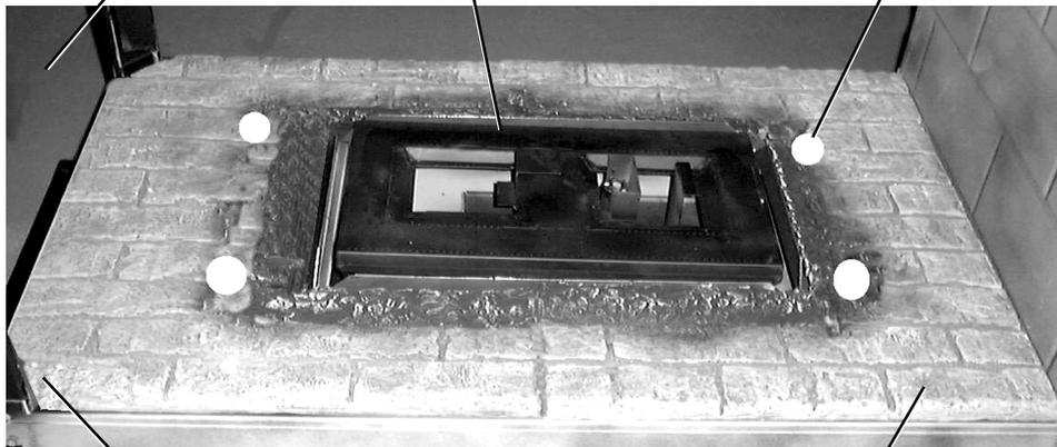
Chamfer Corner Pointing Toward Small Door Opening
