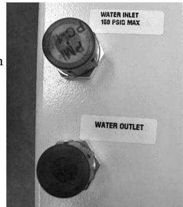
Figure 5-2. Inlet/Outlet Fittings
