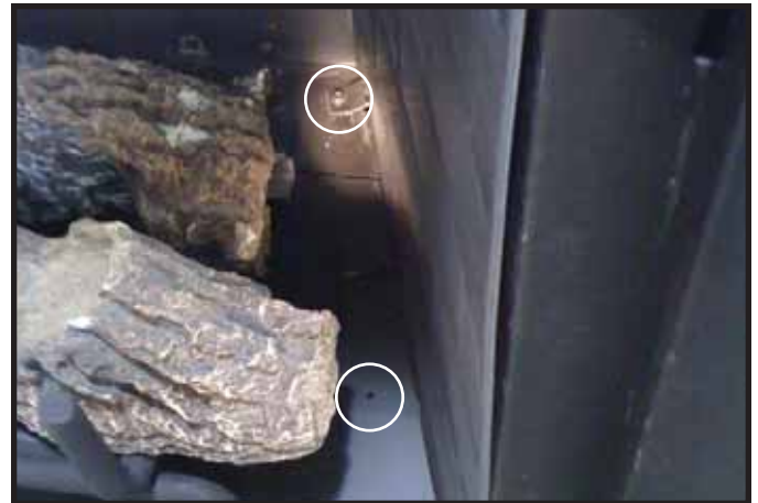
Figure 3.5 Bottom Screws For Metal Refractory
