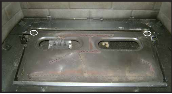
Figure 3.8 Remove Screws from Burner Assembly Rear Corners
