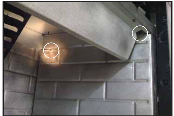
Figure 3.6 Top Screws For Metal Refractory
