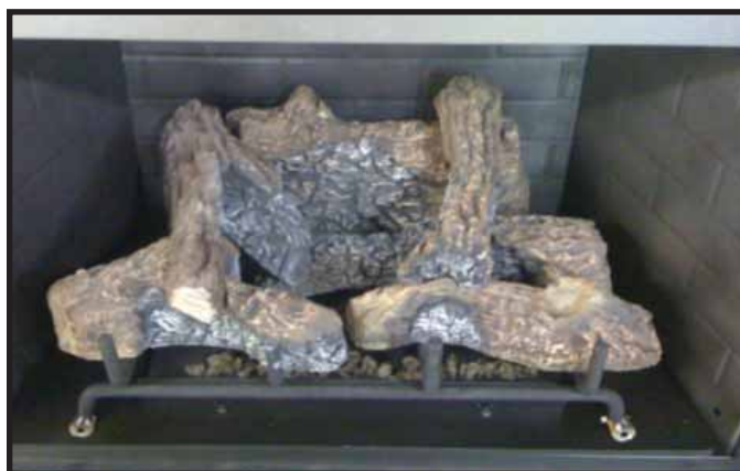
Figure 4. Left and Right Log in Proper Position
