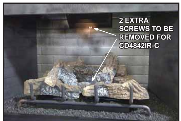
Figure 3.7 CD4842IR-C Extra Metal Refractory Screws
