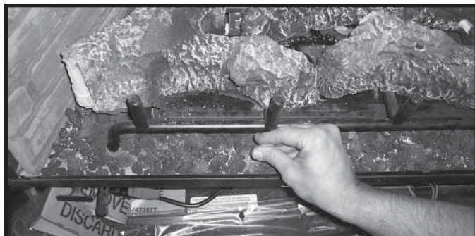
Figure 14.4 Placement of Vermiculite
