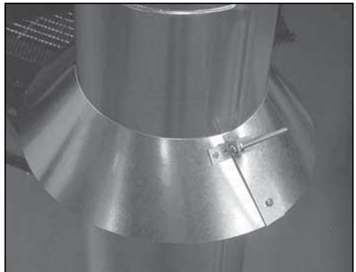
Figure 10.14 Assembling the Storm Collar Around the Pipe
