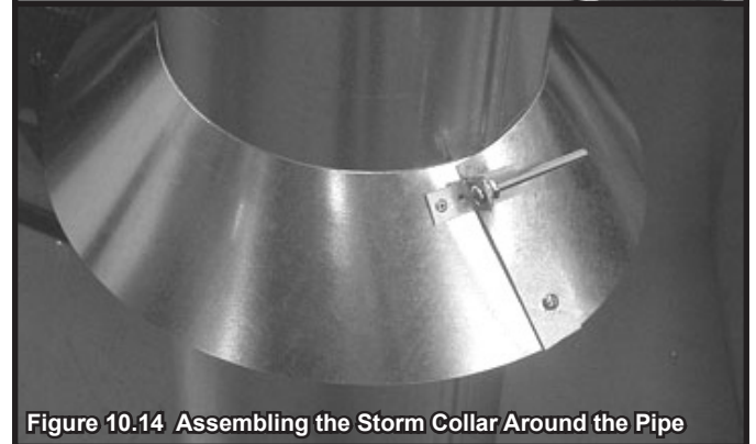
Figure 10.13 Assembling the Storm Collar
