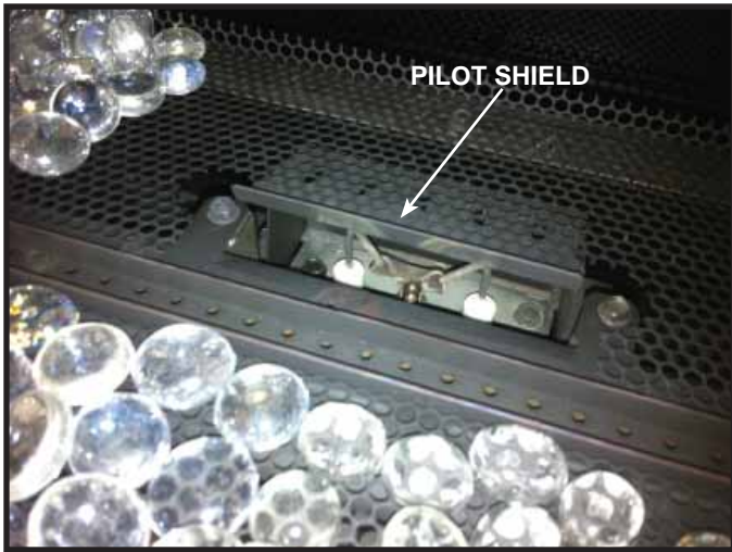
Figure 14.3. Placing Glass Rock Media on Pilot Shield
