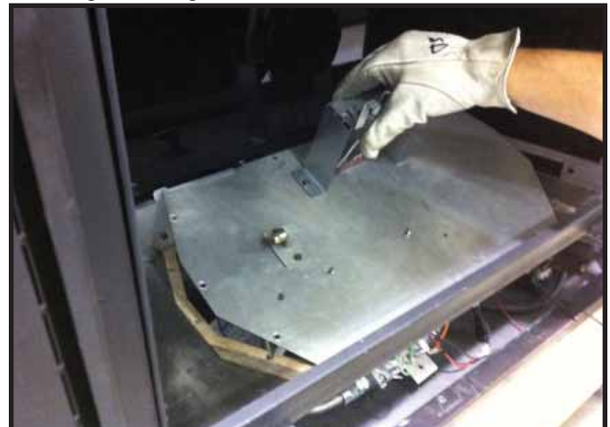
Figure 11.3. Remove Valve Plate
