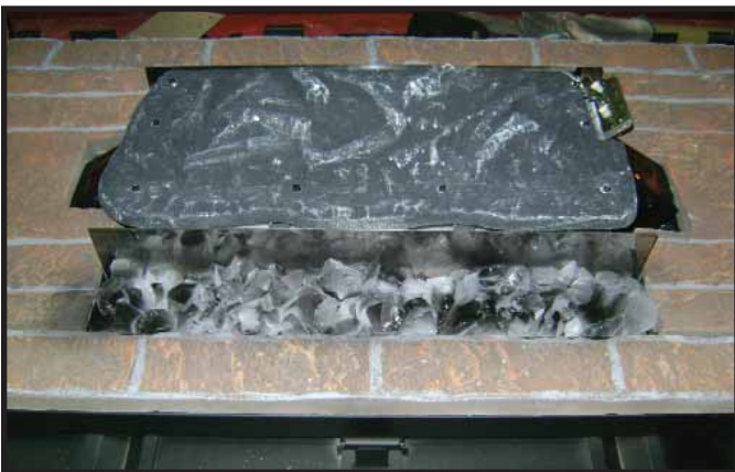
Figure 14.21 Finished Ember Bed
