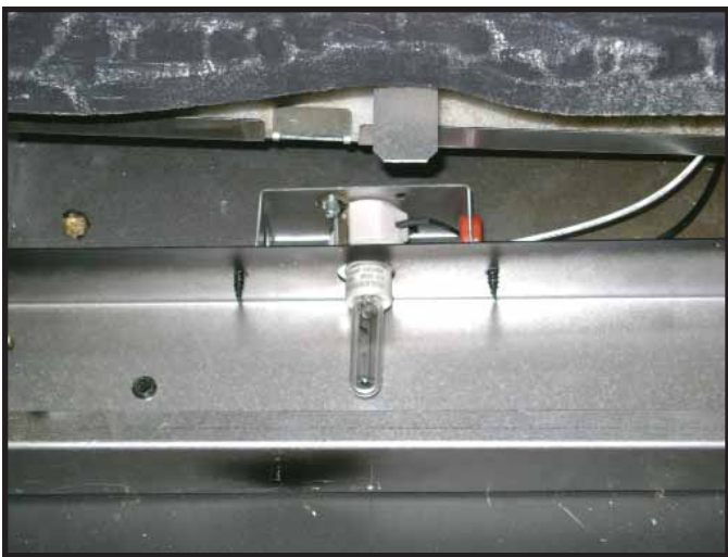
Figure 14.10 Ember Light Bulb Installed
