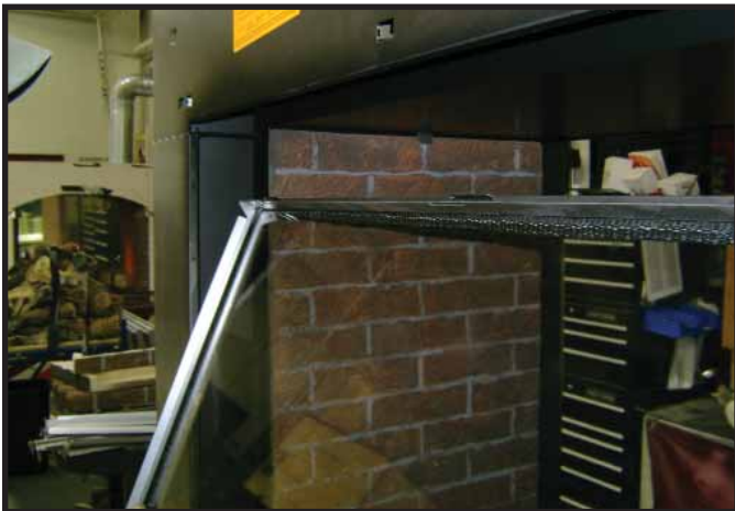
Figure 14.2 Initial Positioning of Frame into Opening.
