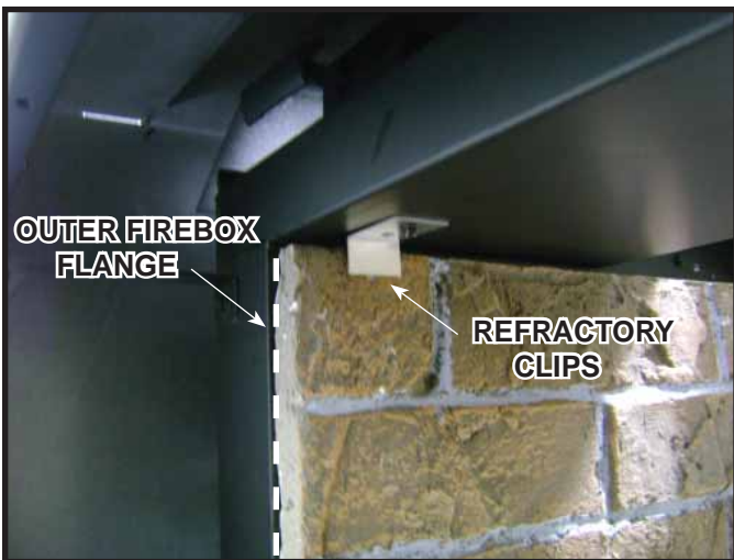
Figure 14.15 Refractory Clip Installation
