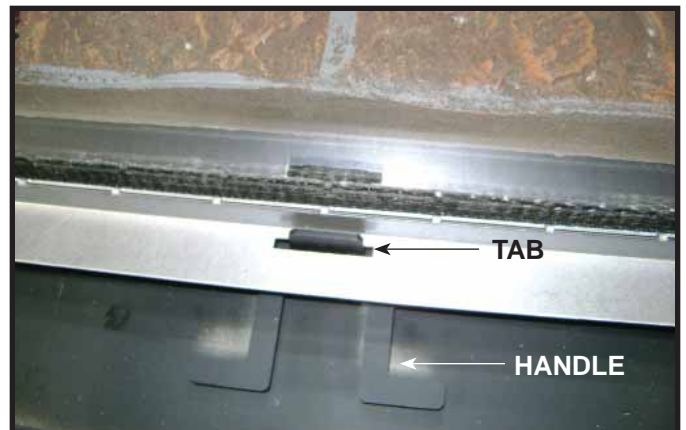
Figure 14.4 Glass Latch Engaged into Frame Latch.
