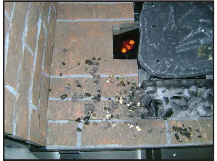
Figure 14.22 Ember Placement on Base Refractory
