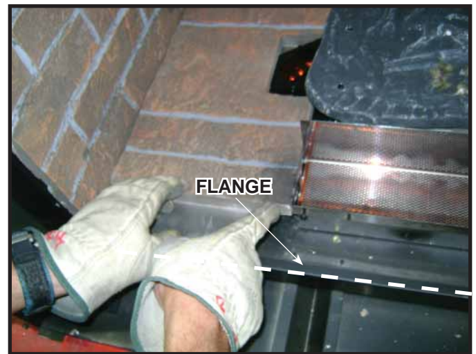
Figure 14.17 Positioning Left and Right Middle Base Refractory
