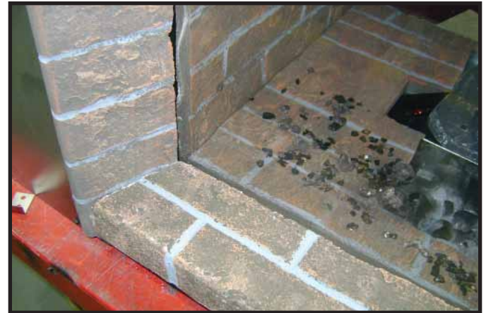
Figure 14.27 Outer Hearth Installation
