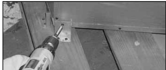
Figure 7.6 Removing Shipping Brackets
