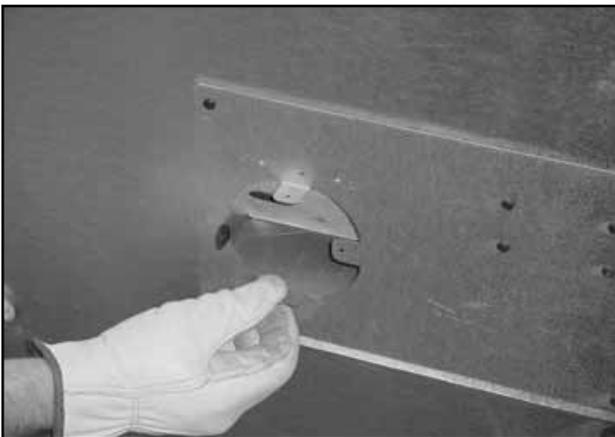
**Figure 7.20 Bending Tabs on Outside Air Kit Collar**
