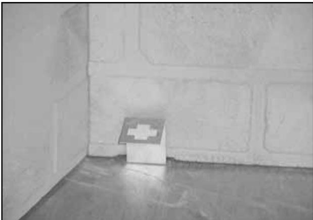
Figure 7.16 Grate Retaining Bracket in Place
