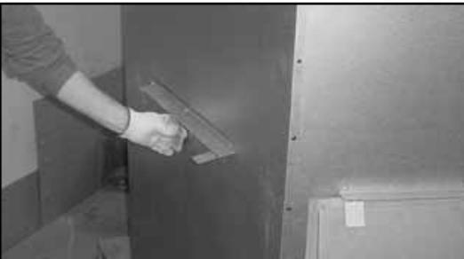
Figure 7.2 Bend Refractory Brackets Back Down
