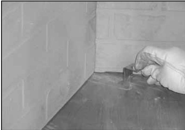
Figure 7.15 Slide Grate Retaining Bracket into Notch
