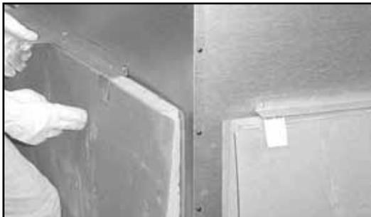
Figure 7.1 Unpack Back Refractory
