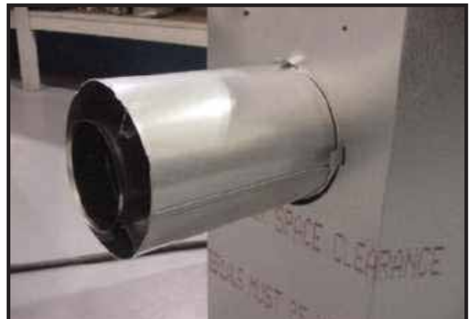
Figure 9.12 Attach the first vent section (it will snap into place). Slide the insulation gasket onto the vent section, up against the appliance and over the tabs.
