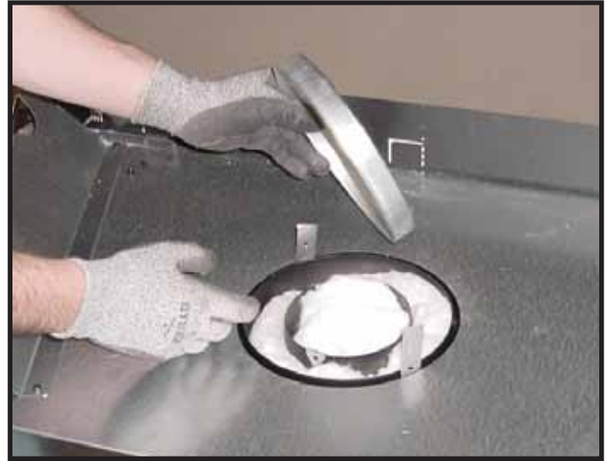
Figure 9.4 Remove the seal cap.
