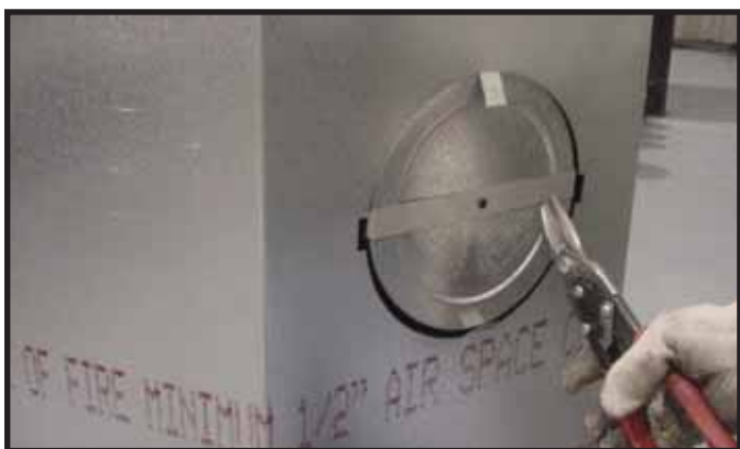
Figure 9.9 Cut the metal retaining band and fold the sides out.
