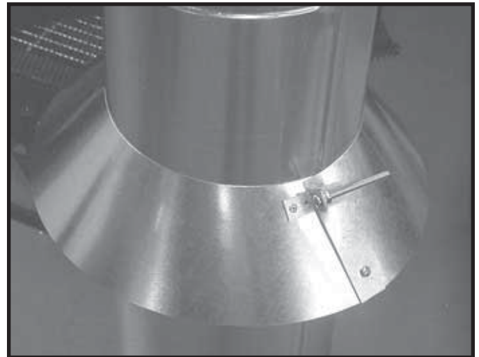
Figure 8.18 Assembling the Storm Collar Around the Pipe
