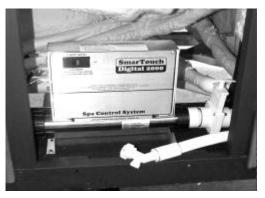
Typical Control &GFCI Slide Valve & Drain Faucet
