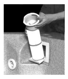
garden hose with a pressurized nozzle push water from the inside to the outside of the filter pleats forcing all trapped particles out. If the filter is far too dirty to be cleaned as described above, obtain from your dealer filter cleaner material. Soak the filter overnight, then hose it down. Filters will last many years if properly maintained.
