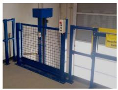
Additional electrical safety-lock for fixing on existing on-site door (to connect the door to the lift-steering)
