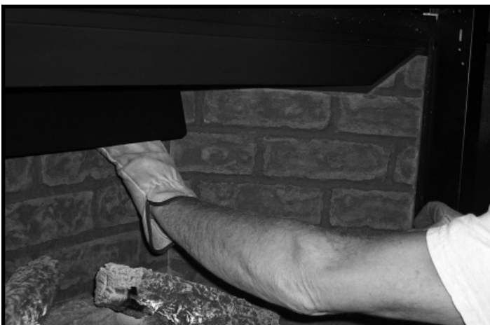
Figure 9 Set Side Refractory in Place
