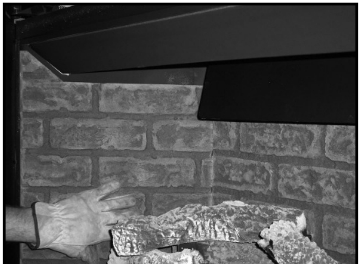
Figure 11 Install Other Side Refractory
