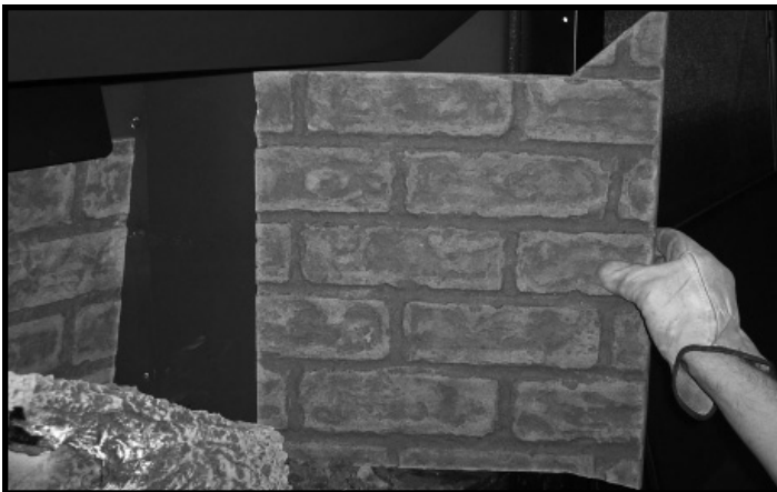
Figure 8 Position Side Refractory
