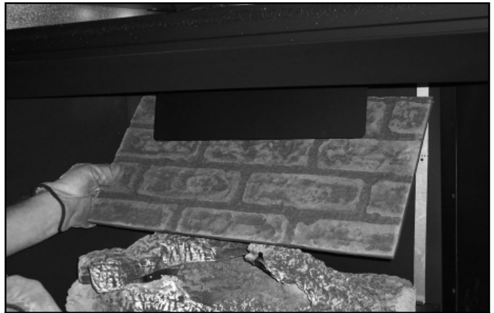
Figure 5 Position Back Refractory for Placement
