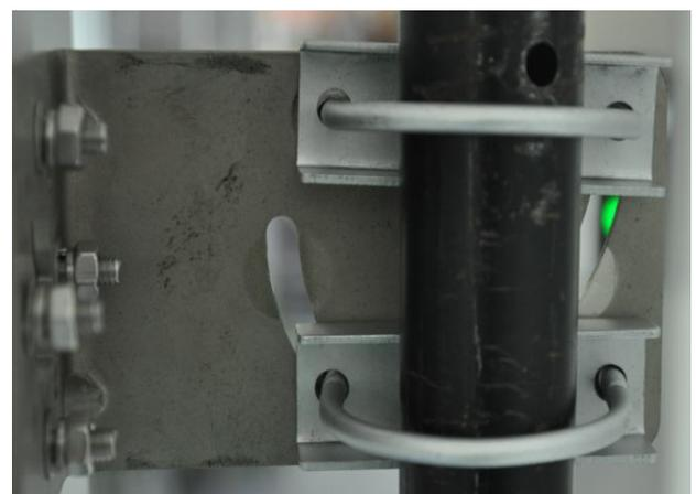
Network bridge is fixed by standard U snap and L angle iron.
