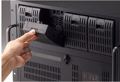
Figure 3.3: Replacing the cooling fan
