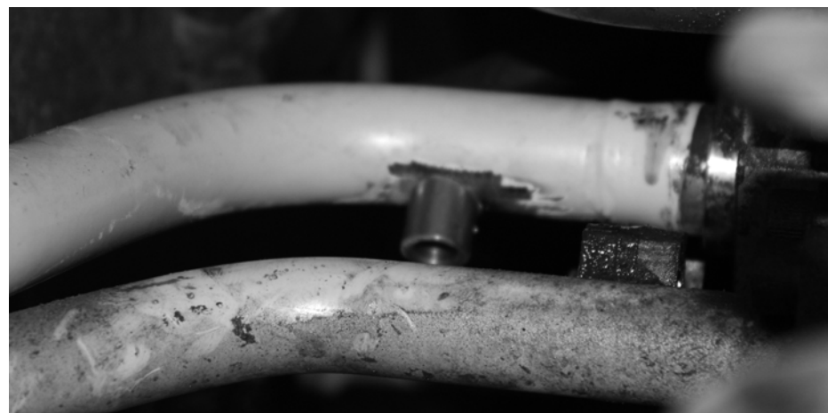
Figure 1-10. Flange Welded to Hydraulic Line at Desired Angle
