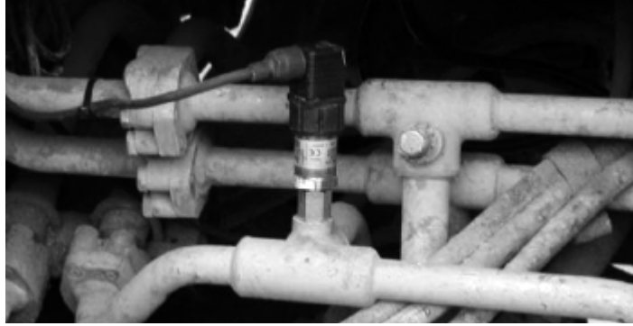
Figure 1-11. Sensor Mounted at Non-Recommended Angle
