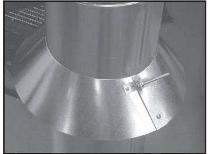
Figure 8.20 Assembling the Storm Collar Around the Pipe
