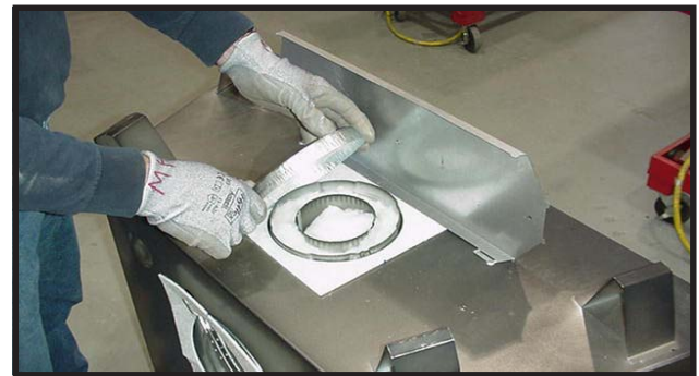
Figure 19. Remove the flue cap.
