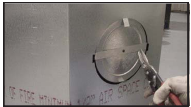
Figure 24. Cut the metal retaining band and fold the sides out.
