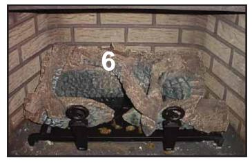
**LOG #6 (SRV340-705):** Place log #6 across log #1 and log #5. The notch in the bottom of log #6 rests in the carved out section on top of log #5 and the left end of the log sits in the horizontal carved out section of log #1.
