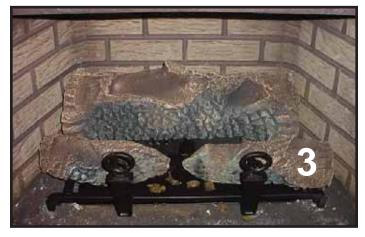
**LOG #3 (2020-142):** Position log #3 by locating its slot over the tab on the front right of the burner. The slot in the right end of the log slides over grate. Slide log all the way back on tab and grate.
