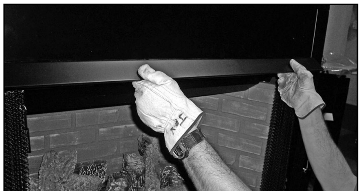
Figure 12.13 Installing the Hood
