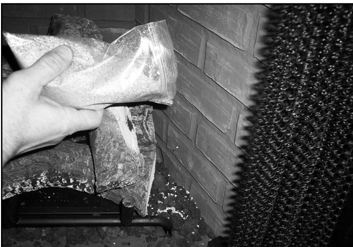
Figure 12.5 Placement of Vermiculite
