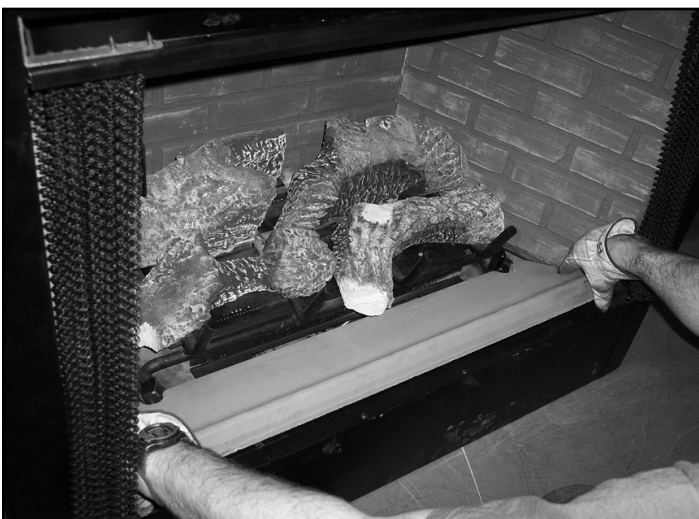
Figure 12.10 Remove Hearth Refractory - Step 1
