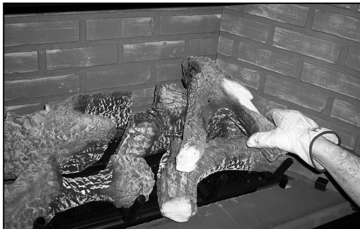
Figure 12.2 Placing Right Top Log
