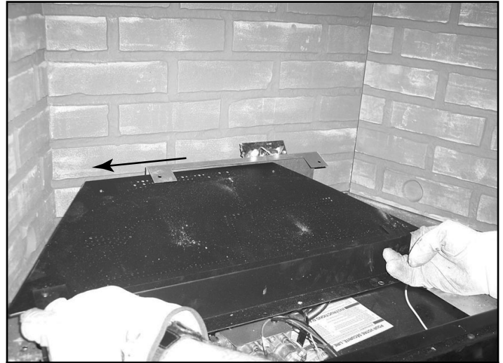
Figure 12.18 Side Burner Assembly to Left
