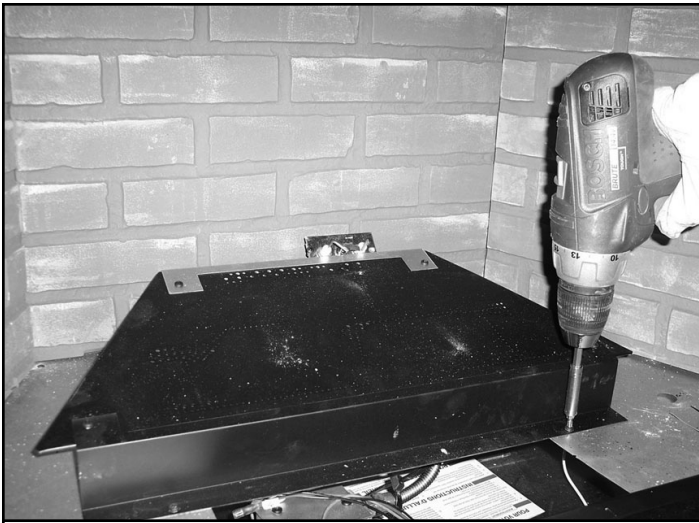
Figure 12.16 Remove Screws Attaching Front Burner Support
