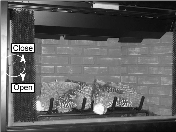
Figure 7.3 Outside Air Kit Handle Location
