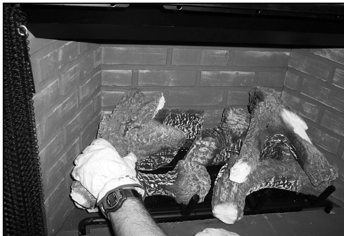
Figure 12.3 Placing Left Top Log
