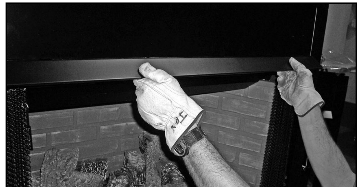
Figure 13.2 Remove the Hood
