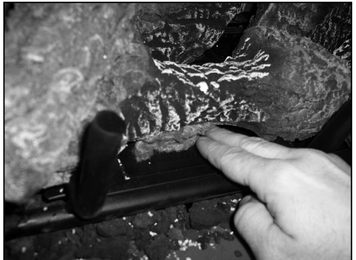
Figure 12.7 Placement of Rockwool Under Front Logs
