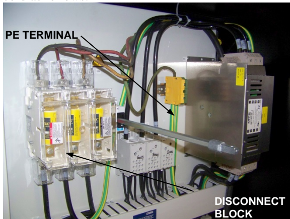
Figure 1-8, Electrical Connection
