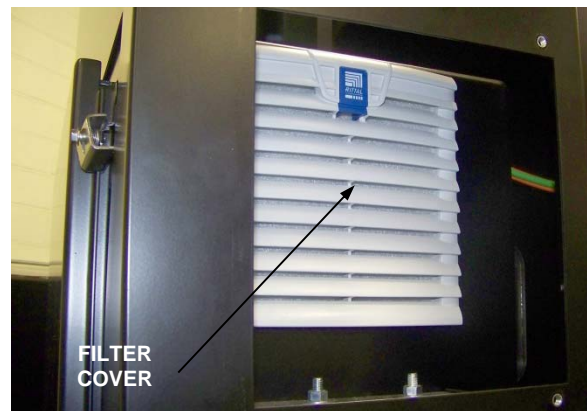
Figure 4-4, Air Filter Cover
