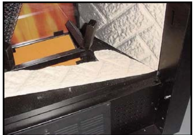
Figure 9 - Hearth Refractory Going In (right side shown)
