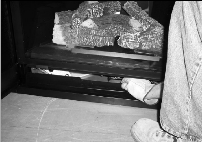
Figure 12.10 Installing Floor Cover
