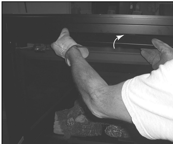
Figure 12.9 Installing Hood
