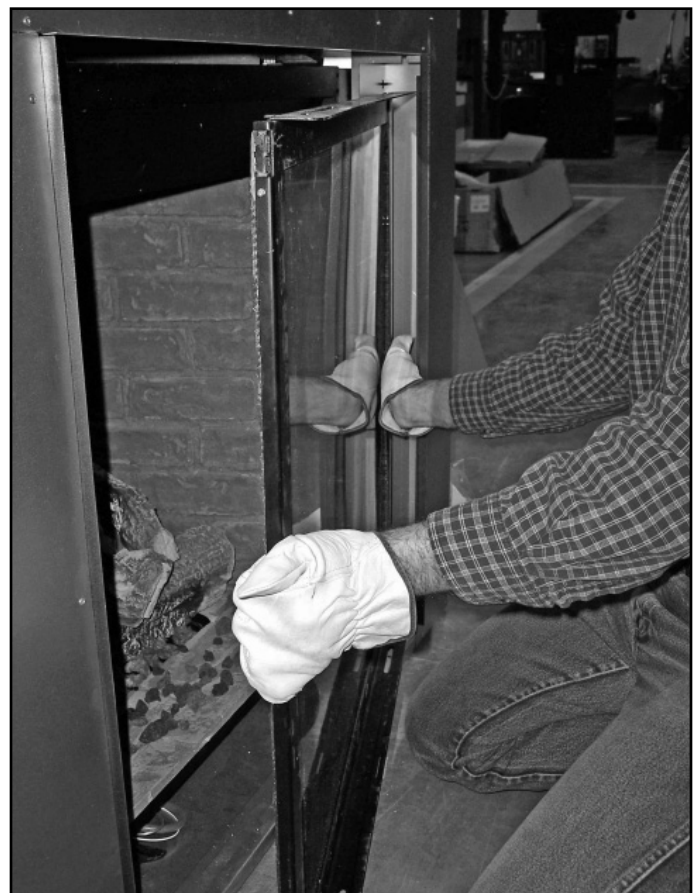
Figure 12.10 Remove Left Side of Glass Frame First
