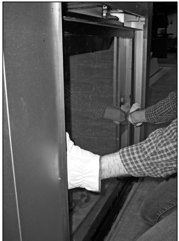
Figure 12.9 Lift Glass Frame Assembly Forward
