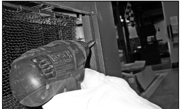
Figure 12.15 Install Refractory Shields
