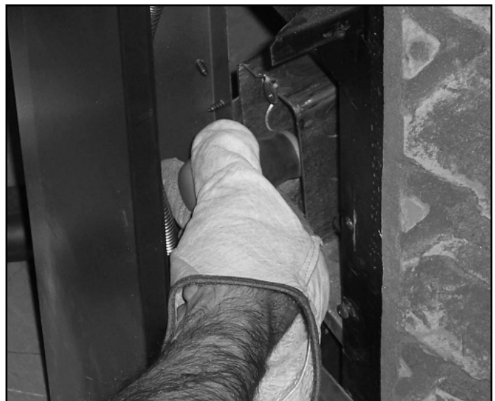
Figure 12.4 Remove Two Screws Holding Junction Box
