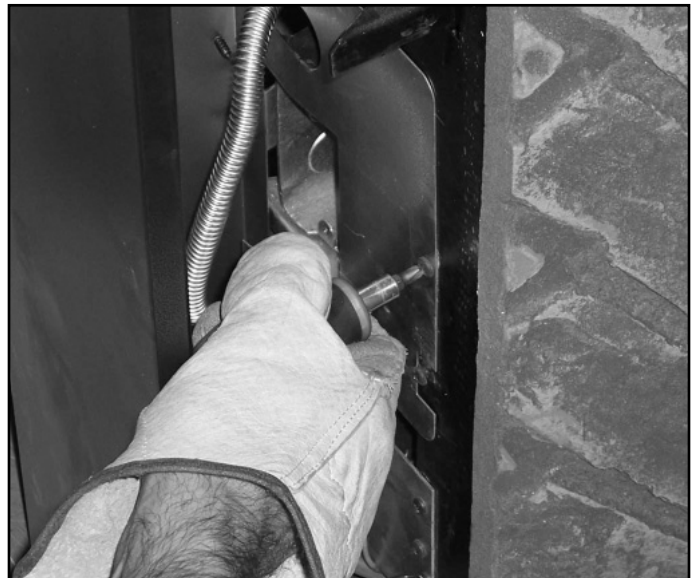
Figure 12.3 Remove Access Panel Screw
