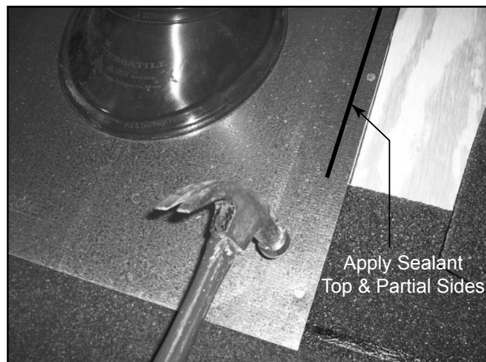
Figure 10.18 Slide Flashing Down, Secure & Apply Sealant
