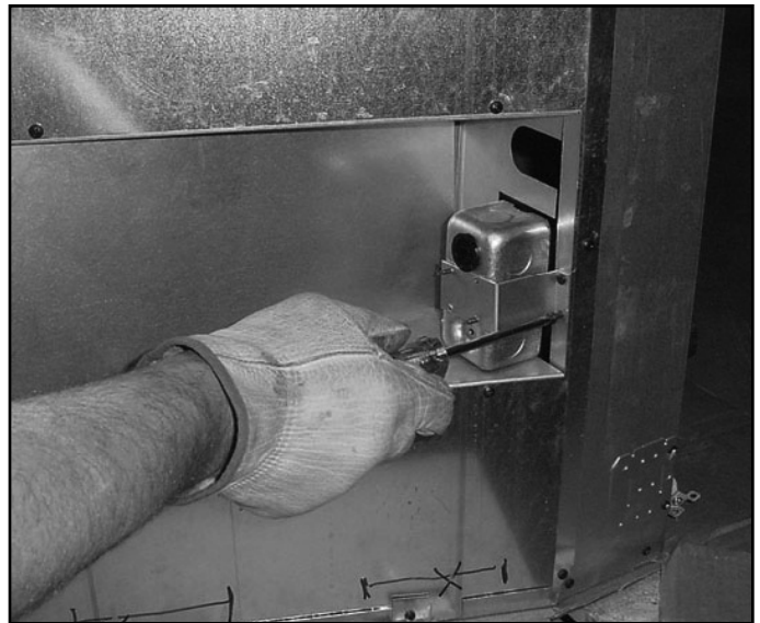
Figure 12.2 Remove Two Screws From Bracket
