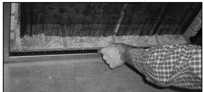
Figure 12.22 Placing Bottom Front Hearth Refractory
