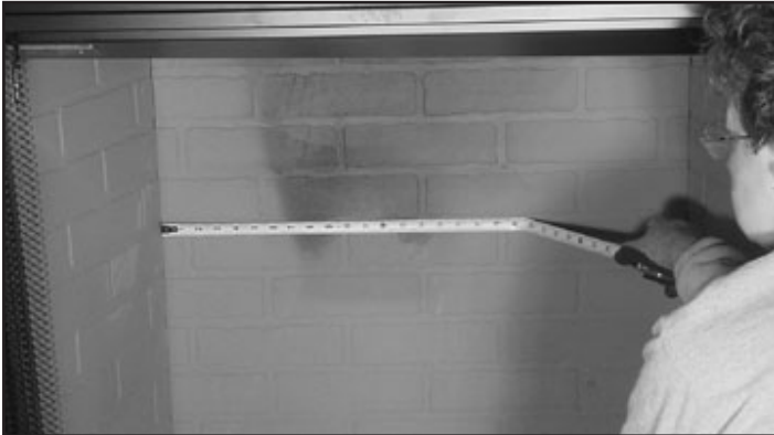
Figure 1 Measure Firebox
