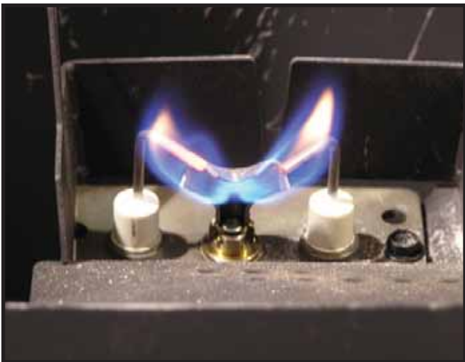
Figure 3.2 IPI Pilot Flame Patterns
