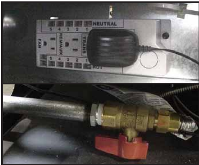
Figure 13.5 Preparation to Install Splatter Guard
