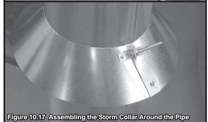
Figure 10.16 Assembling the Storm Collar
