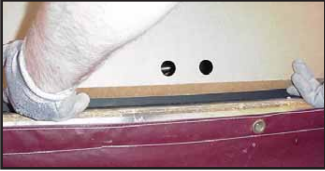
Figure 13.6 Folding Bottom Flap
