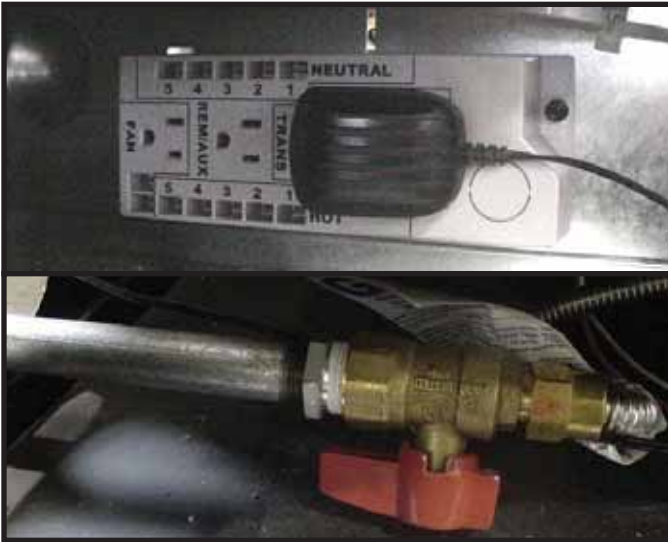
Figure 13.1 Preparation to Install Splatterguard
