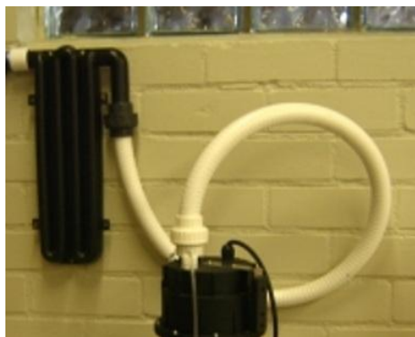
Safety loop (left) to prevent water coming in the airpump
