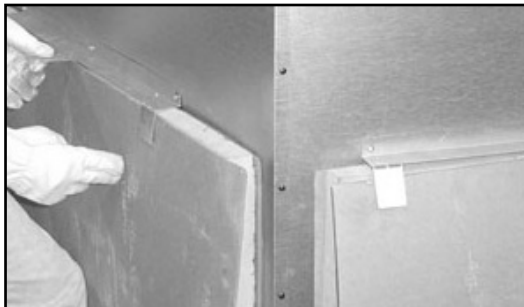
Figure 7.1 Unpack Back Refractory
