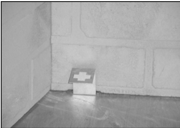
Figure 7.16 Grate Retaining Bracket in Place
