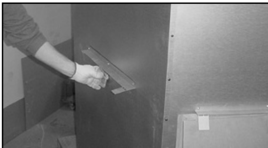
Figure 7.2 Bend Refractory Brackets Back Down
