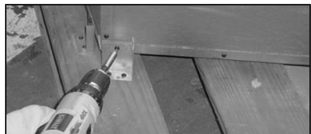
Figure 7.6 Removing Shipping Brackets
