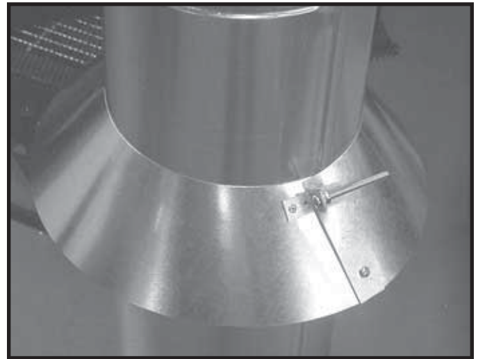
Figure 8.17 Assembling the Storm Collar Around the Pipe
