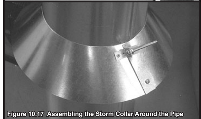
Figure 10.16 Assembling the Storm Collar
